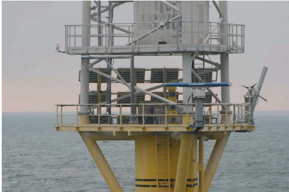
Horizontal and vertical radars as positioned on the metmast in the OWEZ wind farm area. Photo: M. Poot.
